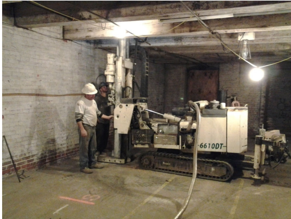
Photograph 3. Geoprobe equipment for performing borings- rubber tracked.
