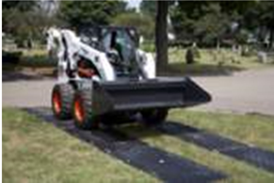
Photograph 2. Mats to be used to protect the ground surface.
